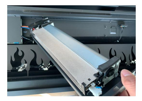
**Step 2** Unscrew the screws to disconnect the heater from the heat assembly. Unplug and replace.
